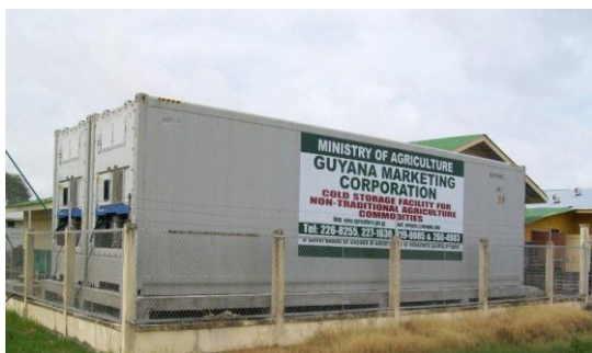
Cold Storage Facility at Central Packaging Facility
