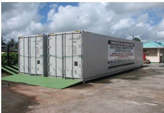
Cold Storage Facility at Parika Agro Packaging Facility
